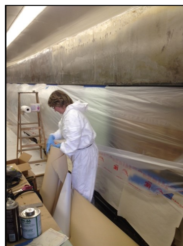
Tylene Crouch is putting up masking paper in preparation for interior painting.
