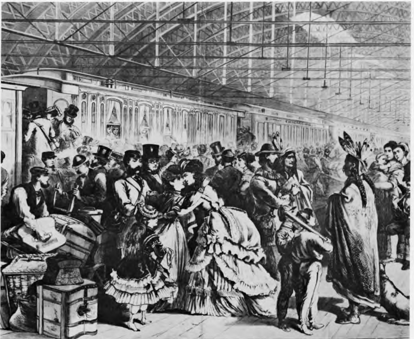
GREAT RAILWAY STATION AT CHICAGO—DEPARTURE OF A TRAIN.
