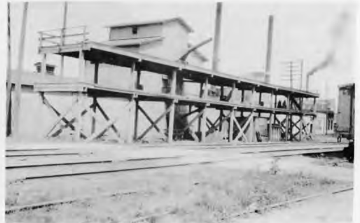
Freeport Terminal Icing Platform.
