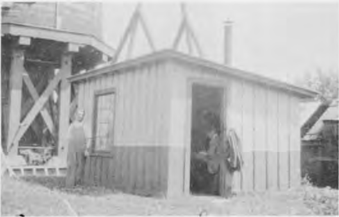
Seward Pump House.
