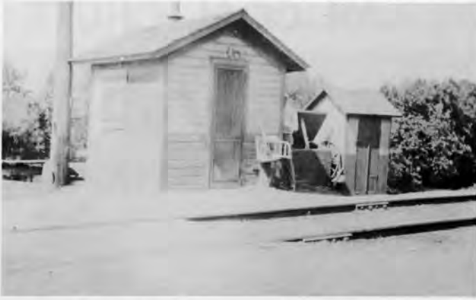
Freeport Terminal Watch house Van Buren St. Valuation photos -ICHS Collection.
