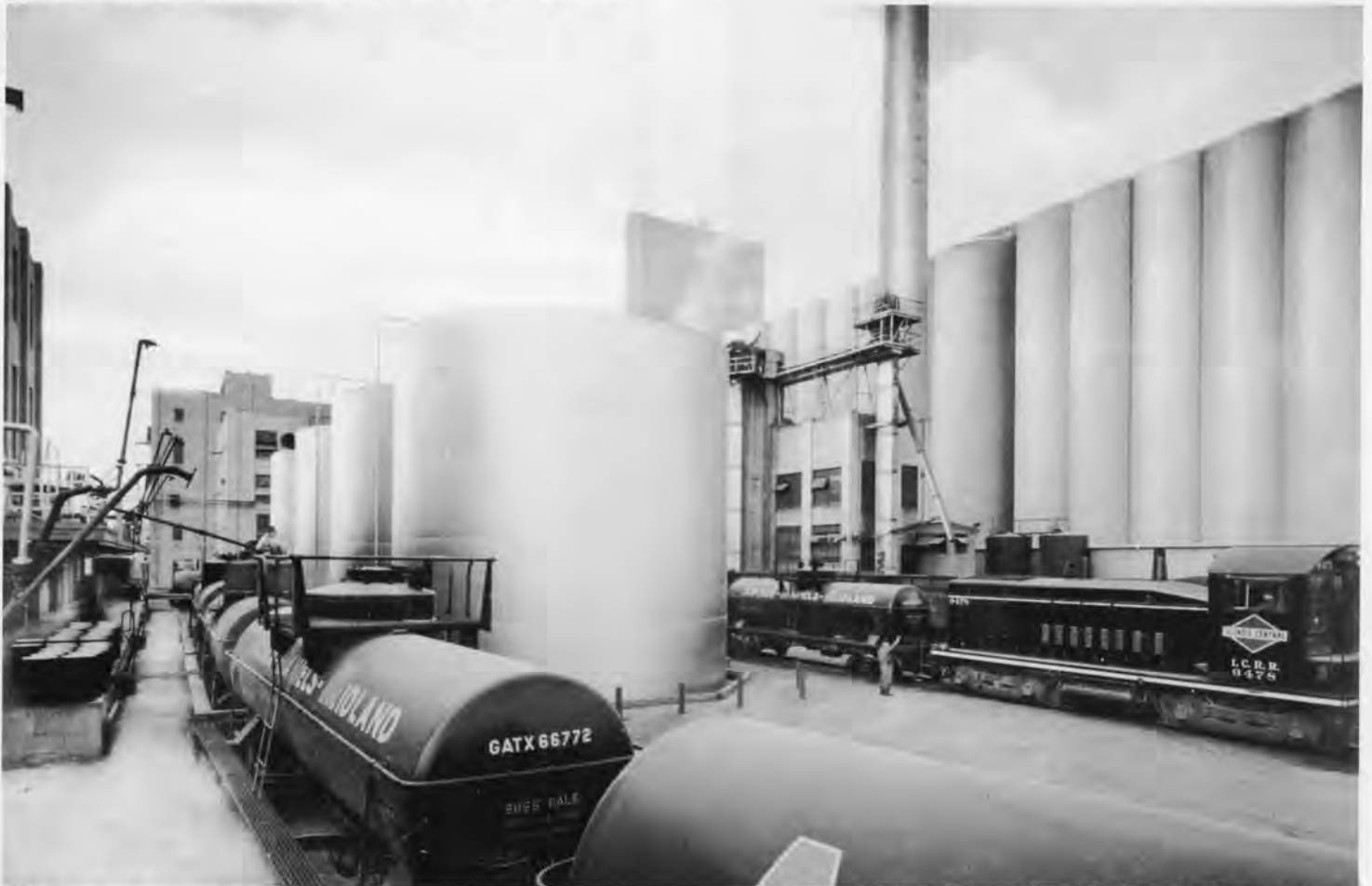
SW 9 # 9478 switches at ADM in the 1950's.
