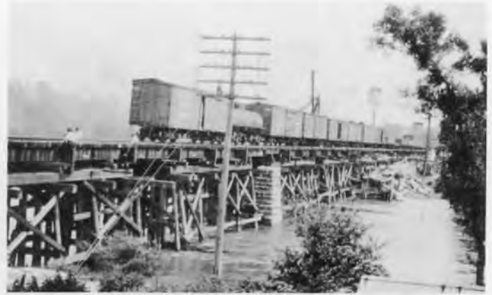
Rockford Rock River - bridge W86.06 under construction. 694' long - 10 spans. Masonry piers built 1887.
