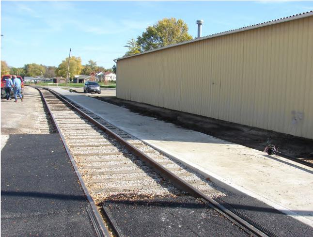
Improvements to benefit our guests has been made with the recent installation of a 280 foot concrete platform between Hamilton and Buchanan Streets, Monticello. This will accommodate the loading of passengers with the addition of equipment on the *POLAR EXPRESS*. Five new additional platform lights has also been installed and placed in service.
