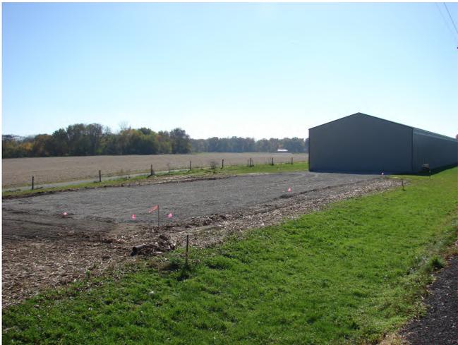
Grading has been completed for the extension of 184 feet of the carbarn, located on the north side of Nelson Crossing. This will increase the car capacity of Tracks 1, 2 and 3 inside the building to house more equipment and provide protection from the elements of weather which can cause equipment and paint to deteriorate. During the Polar Express Season, an entire train can be housed on one track, which will improve operations.
