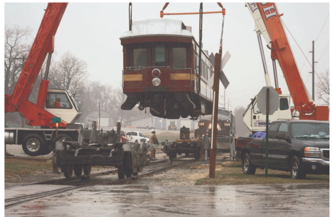
Wabash No.6 dangles from the cranes while Doug Butzow and Paul Bundy prepare to pull the trucks in place under the car at Monticello.
